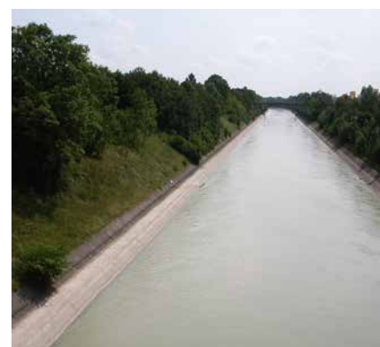
The River Inn, north-west from Mühldorf am Inn. A canal is characterised, inter alia, by an absence of a connection from the body of water to the floodplain or foothills, and limited variation in flow behaviour.
