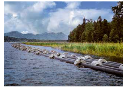
Temporary storage of the ready-to-lay pipes for the Chiemsee perimeter sewer system. Perimeter wastewater treatment systems are laid mostly on land, but partially also under water.
