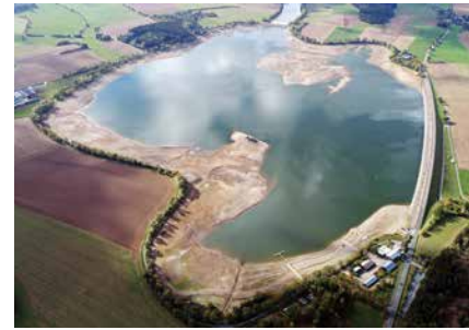
The Förmitz Dam with dry river banks in September 2018
