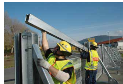
Test set-up of mobile flood defence elements in the town of Miltenberg
