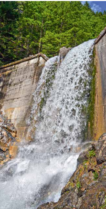
It is not very pretty, but technical measures, like the mudslide barrier here on the Faltenbach stream near Oberstdorf in the Oberallgäu rural district, protect residents from the dangers of an alpine torrent.
