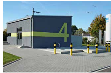
System for removing trace substances at the wastewater treatment plant in Weissenburg
