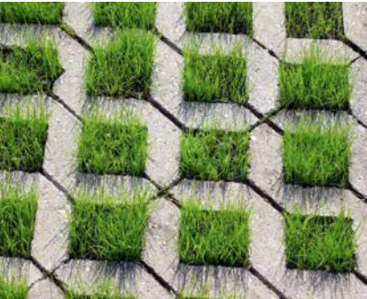
Precipitation water does not always have to be routed into the sewer system. Permeable structural elements enable seepage.
