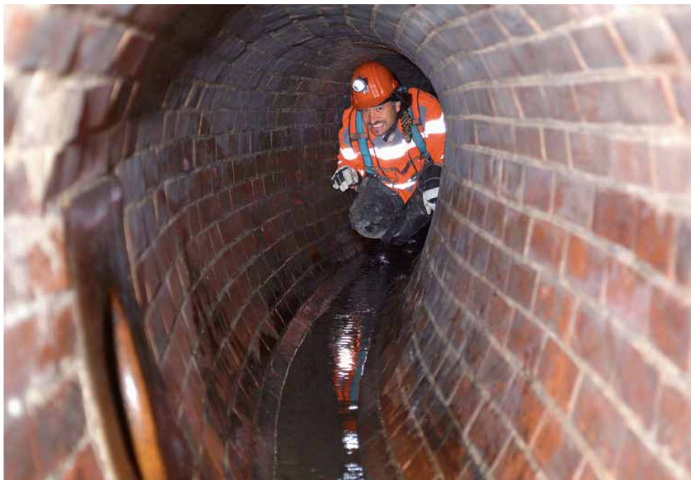
The condition of wastewater collectors with a transverse section is checked by means of a walk-through inspection.
