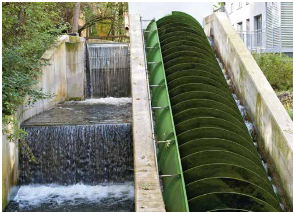
Hydrodynamic screw: Fish-friendly hydropower technology for small developed water volumes; often used to exploit residual water.
