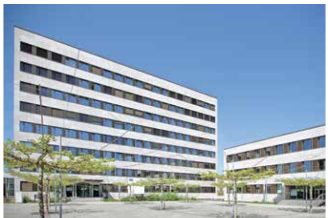
Special program for the energy rehabilitation of government buildings: State Finance Office and State Building Authority Würzburg, co-financed by the European Union out of the European Regional Development Fund (ERDF).
