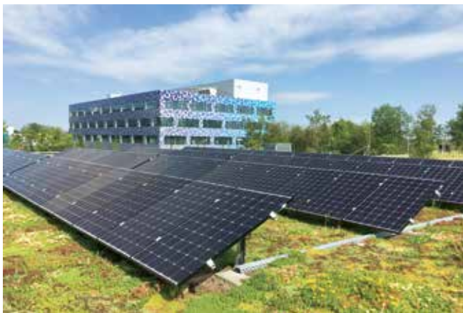
Use of renewable energy in government construction projects: Combination of photovoltaics with green roofs on a building on the Garching research campus.
