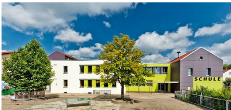
Dürrwangen Primary School, given an energy-efficient refit as part of the second economic stimulus package
