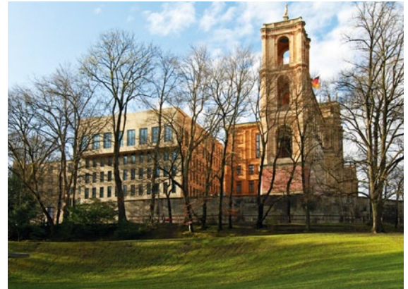
Bavarian State Parliament, extension in the northern court: this building was constructed to passive house standard.
