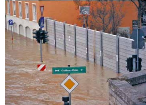
Mobile flood defence units prevent flooding of Würzburg city centre, January 2003.
