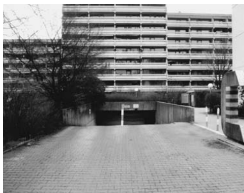
Fig. 21: Example of a not enclosed underground car park ramp
