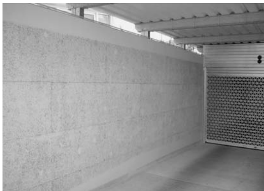
Fig. 26: Inner wall of the underground car park ramp, paneled in an absorbing manner
