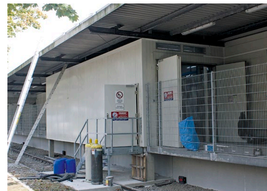
From left to right: the R-723 plant, the central control panel and the entrance to the soundproofed room in which the refrigeration plant is located
