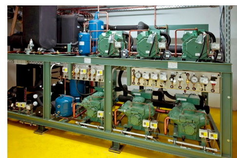
Below: Compressor and control panel Left: Hops mill for the processing of hops at low temperatures
