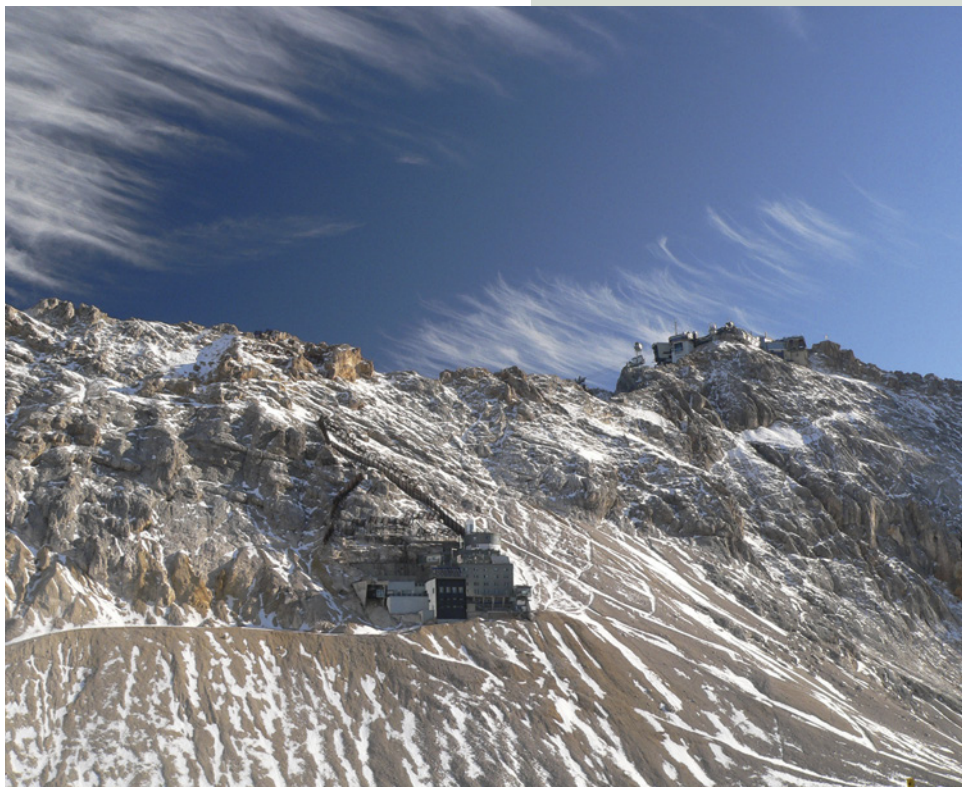
Environmental research station Schneefernerhaus
