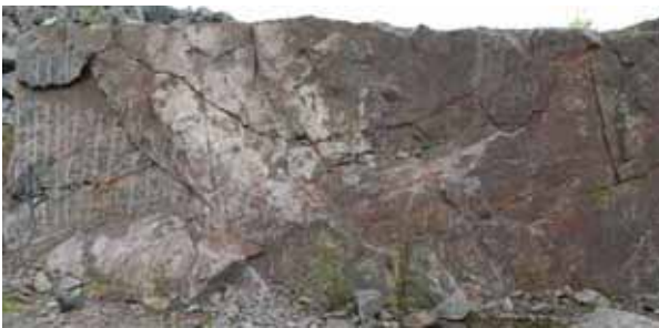
Figure 2 – An example of the walls in the dimension stone quarry. The wall was mapped and photographed.
