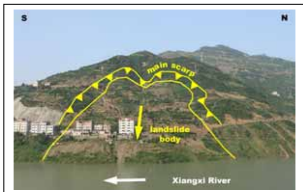
Figure 6 – Inactive landslide near Xiakou Town (water level 155 m). The landslide body was partly stabilised by concrete piles near the buildings.
