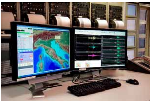
Figure 1 – INGV Seismic Monitoring headquarter
