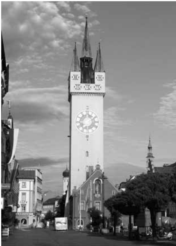
Figure 1 – The Gothic city tower of Straubing, standing on a Pleistocene terrace is a typical building with a combined brick and natural stone construction.
