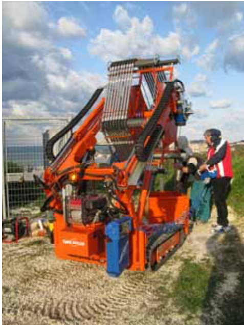
Figure 3 - DMS installation in place
