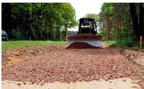
Links: Recycling-Beton
