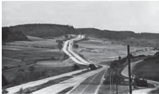
Visually disjointed arcs and tangents (above) versus a continuous, coordinated ribbon (below).
