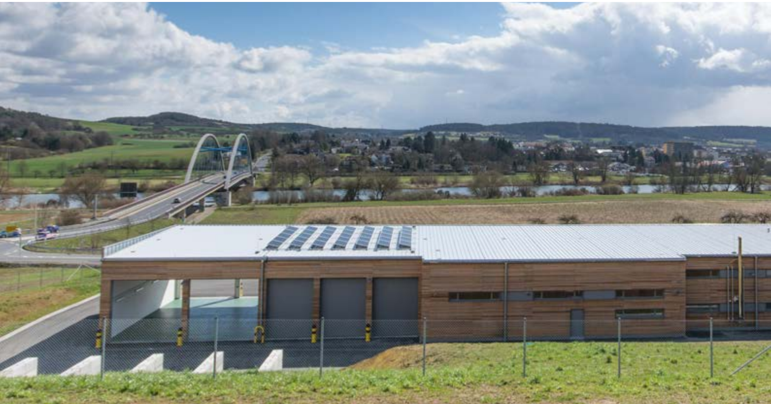
Hafenlohr depot of the Lohr road maintenance service
