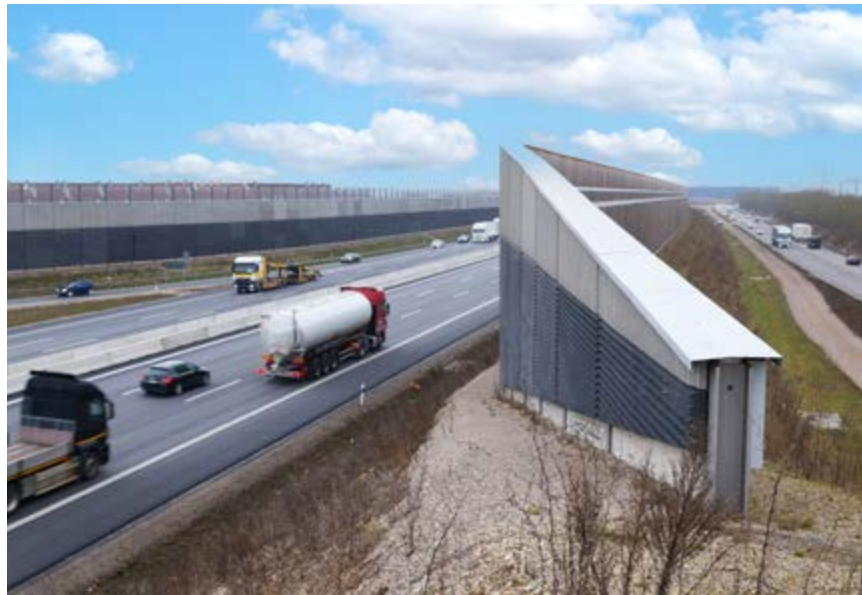
A3, six-lane upgrade south of Regensburg with noise protection
