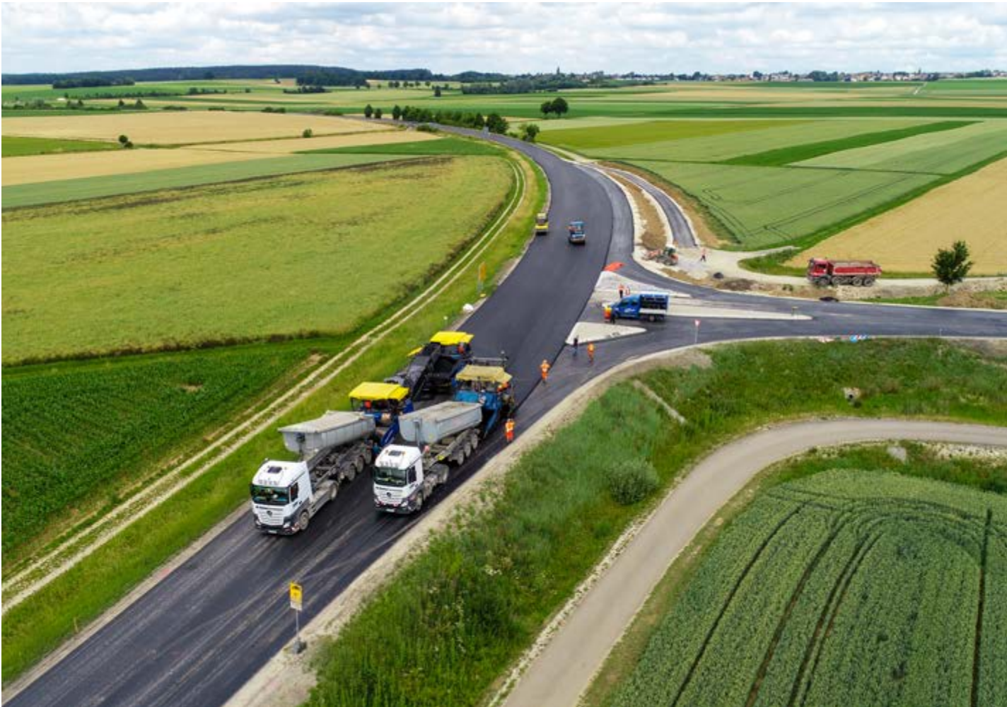
B 13, road resurfacing near Eitensheim
