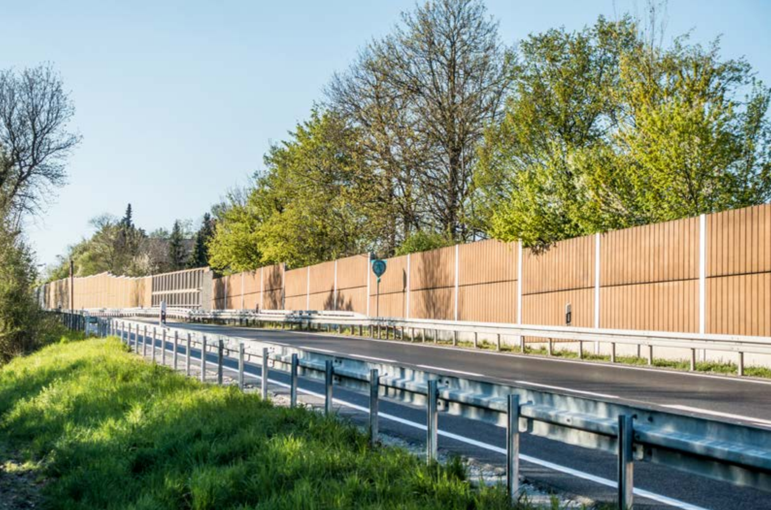
Mitigating traffic noise with a noise barrier
