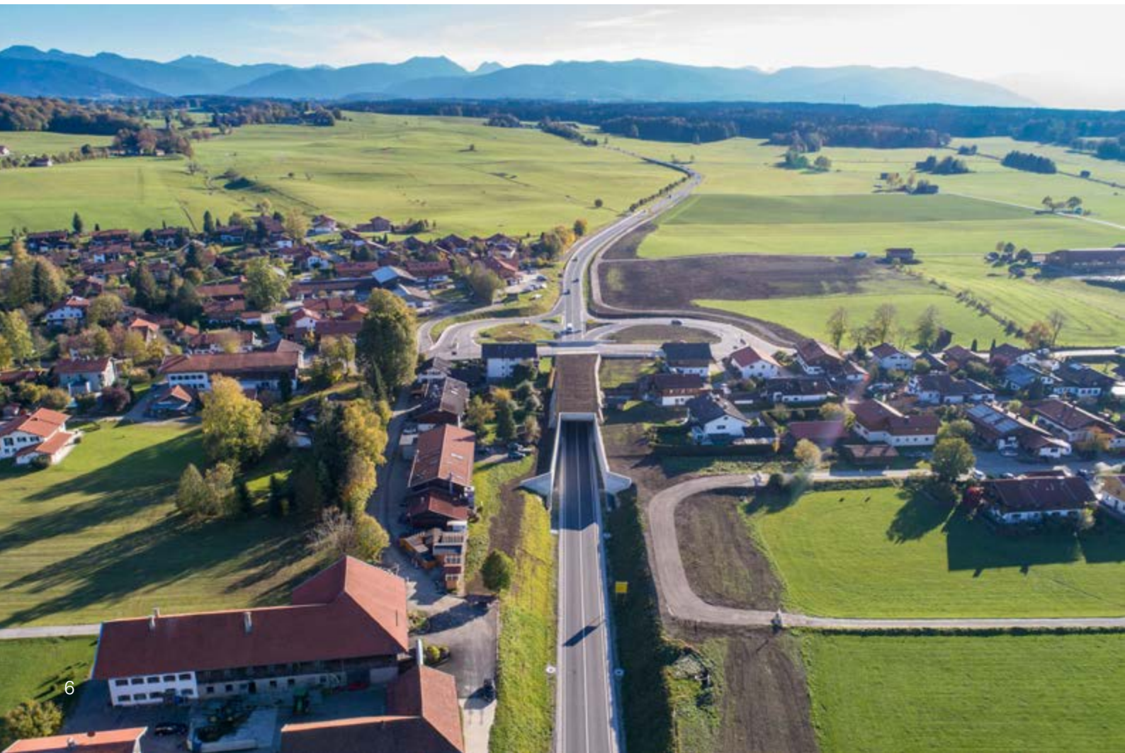
B 318, grade-separated upgrade of the junction with the MB 19 district road in Warngau
