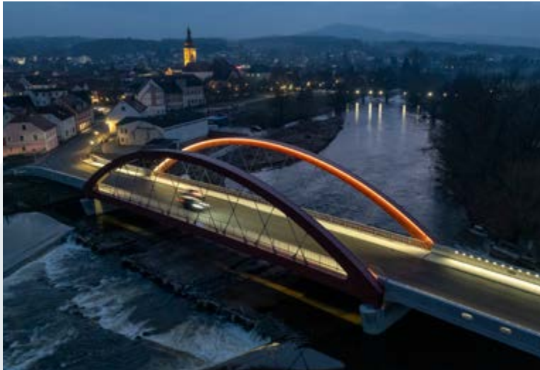
St2145, Modernisation of the bridge over the River Regen at Nittenau
