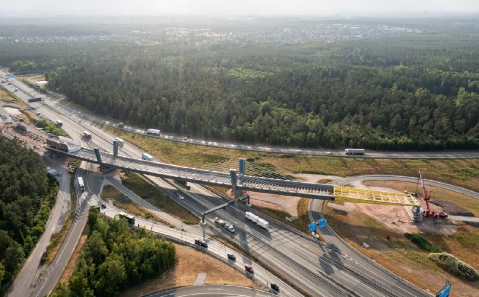
A 6/A 9, Nuremberg-East motorway junction flyover
