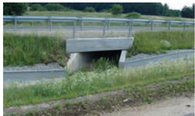
Amphibian guidance devices on the B 470 near Burk between Forchheim and Wimmelsbach
