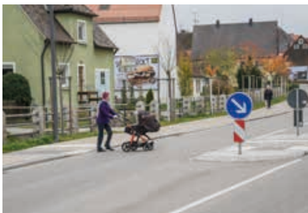
Separate crossing point with kerb and zero drop; tactile floor elements in picture and sketch
