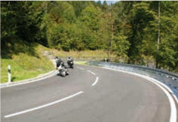
➤ Bend with retrofitted underrun protection
