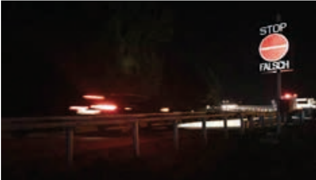
≡ A 9 wrong-way driver warning system
