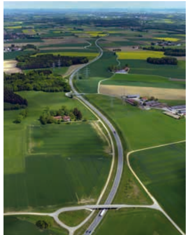
☞ St 2580, airport tangent east in construction phase V; aerial view looking north (Erding)
