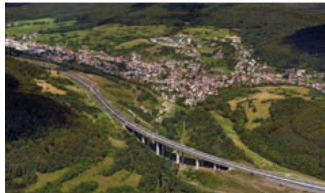
➤ A 3, Kauppen bridge at Waldaschaff; the new route has been moved up to 300 metres
